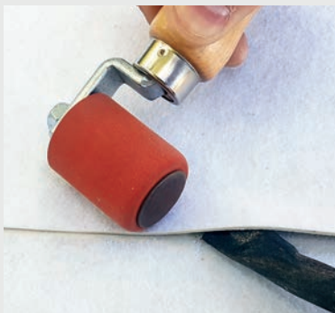
Fig 2: 1½" triple-welded seam
