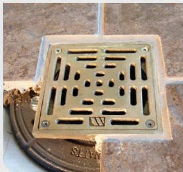
Fig 3: Cast Drain with Nickel-Bronze Strainer
