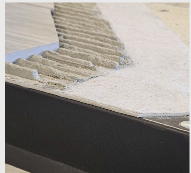
Fig 4: PVC coated flashing
